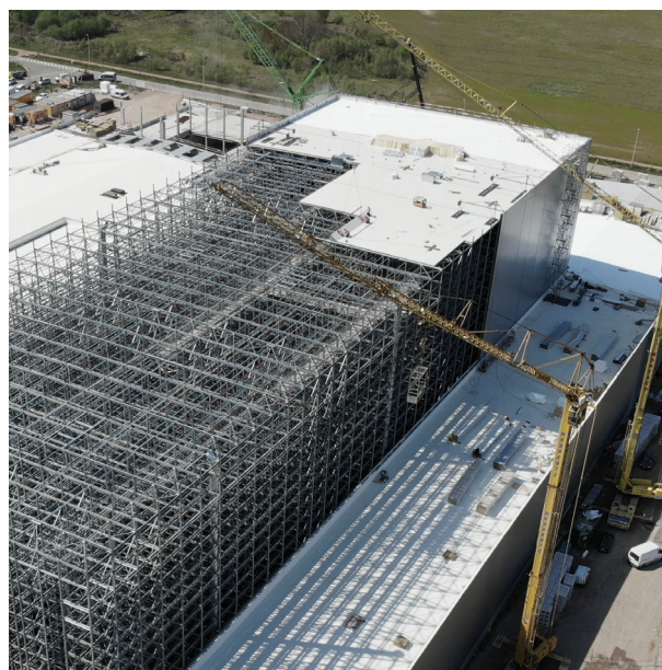
Fig. 15: Flat roof installation
